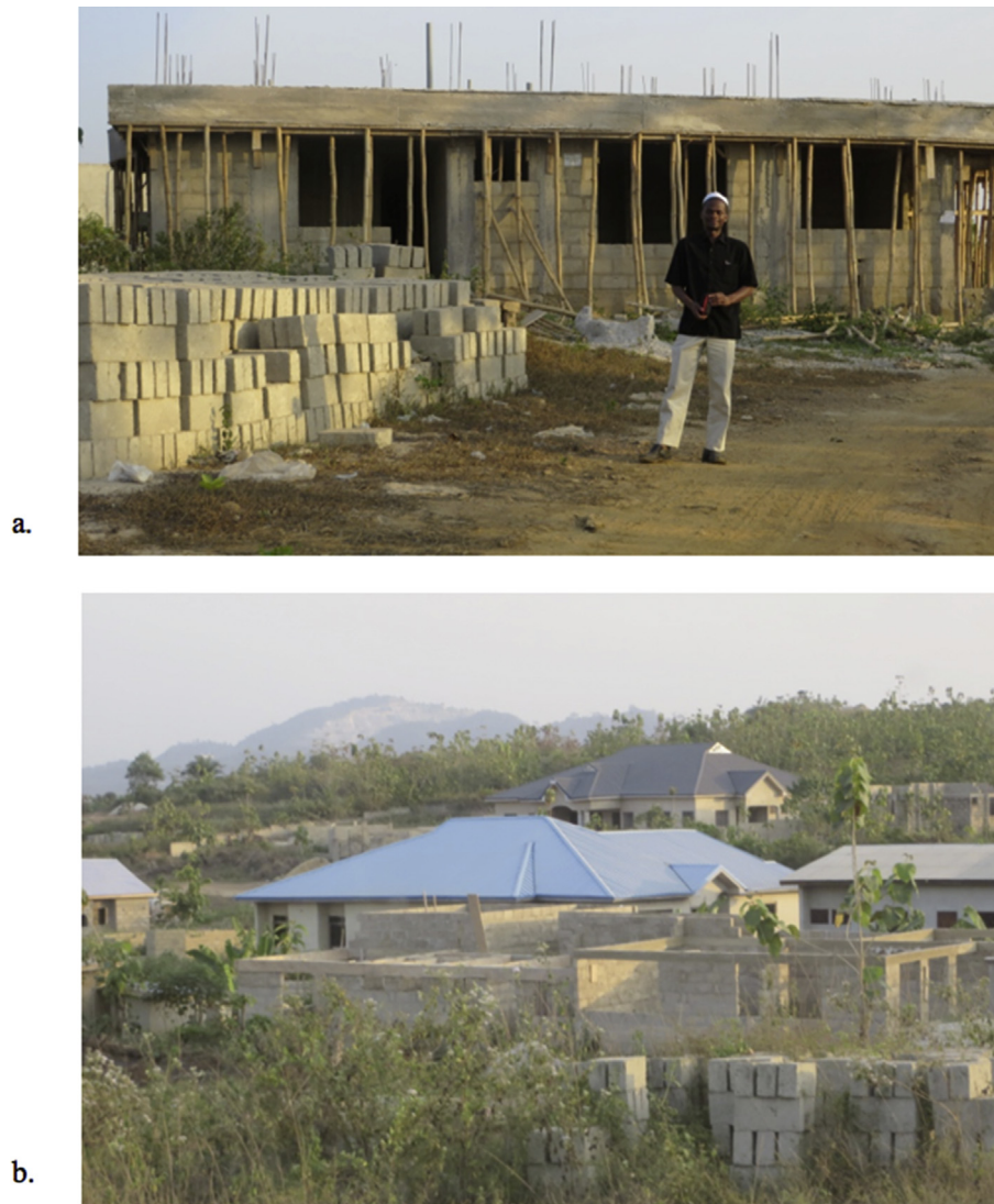
Fig. 8. Ground images from Ghana study area taken February 2014. a. Example of unfinished residential structure, where building can take five to ten years to complete and squatters may reside during various stages of construction. b. Example of large, moderate to high quality residential structures commonly built in the peri-urban areas of Accra and Kumasi.
